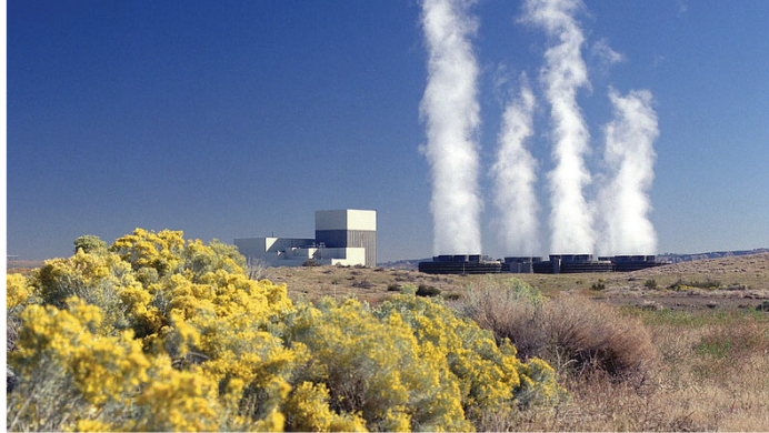
The Columbia Generating Station (Image: Energy Northwest)
